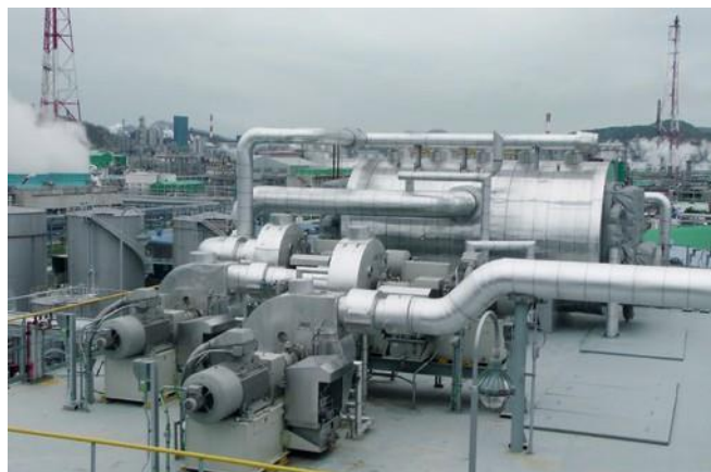
Fig. 4: An Evaporator evaporates water at low pressure
